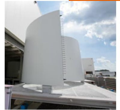
The pre-cast concrete components for the hybrid towers are shipped from the production site near the coast in Osterrönfeld in Schleswig-Holstein via the Kiel canal for the installation of wind power systems in North Germany and Scandinavia.
