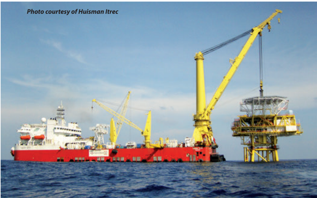
Crane ship SAPURA 3000 placing topside installation
