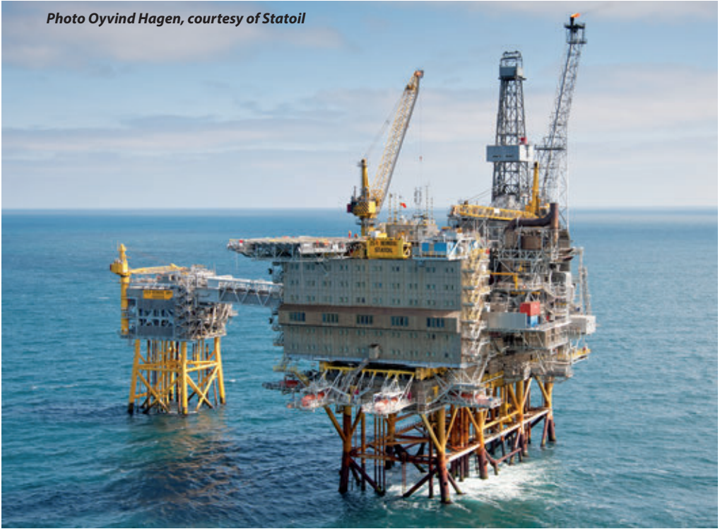
Fixed steel installation on the Heimdal field
