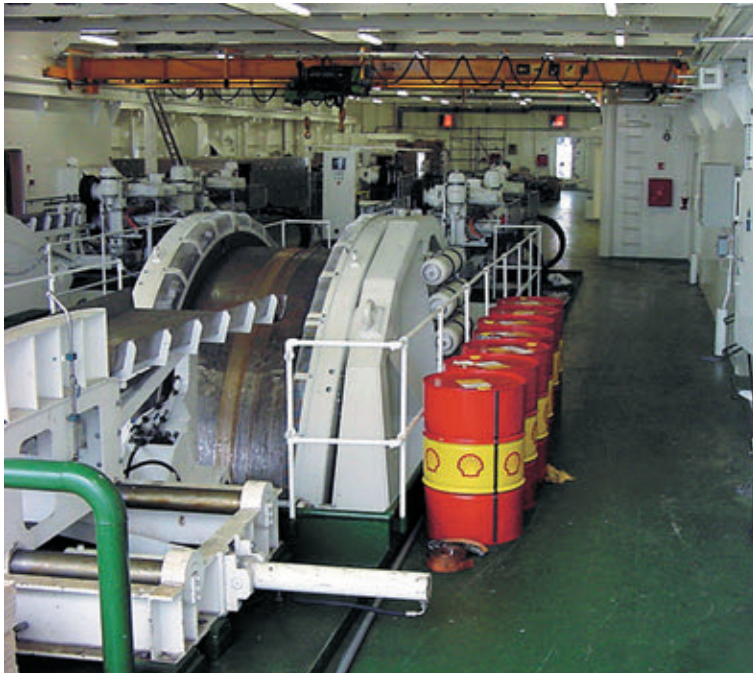
Cable handling machinery of ATLANTIC GUARDIAN
