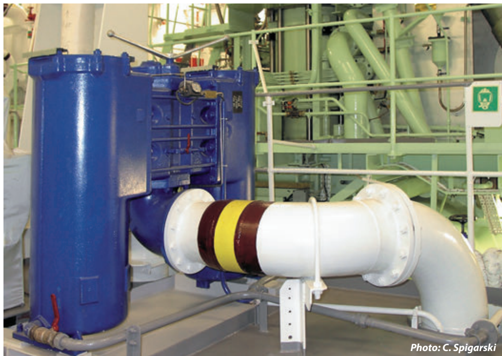
Main Engine fuel oil duplex indicator filter
