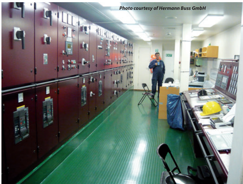
Main switchboard in the Engine Control Room
