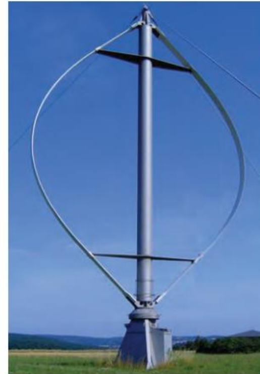
Figure 6.59 Vertical axis wind turbine. (Courtesy of US National Renewable Energy Lab.)
