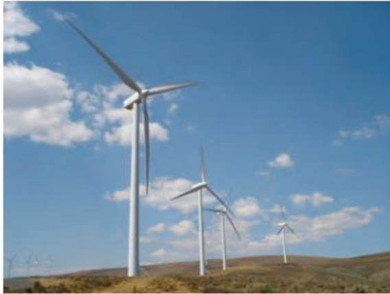
Figure 6.57 Horizontal axis wind turbines.
