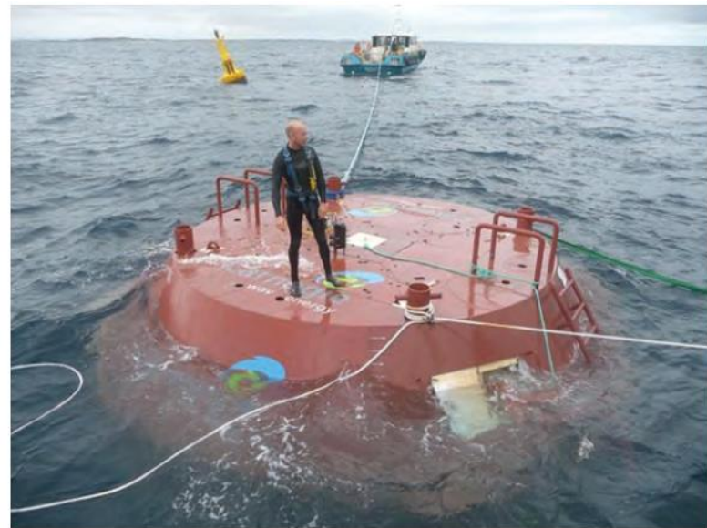
Figure 6.77 Buoyant actuator during the installation. (Courtesy of Carnegie Wave Energy through Wikipedia.)
