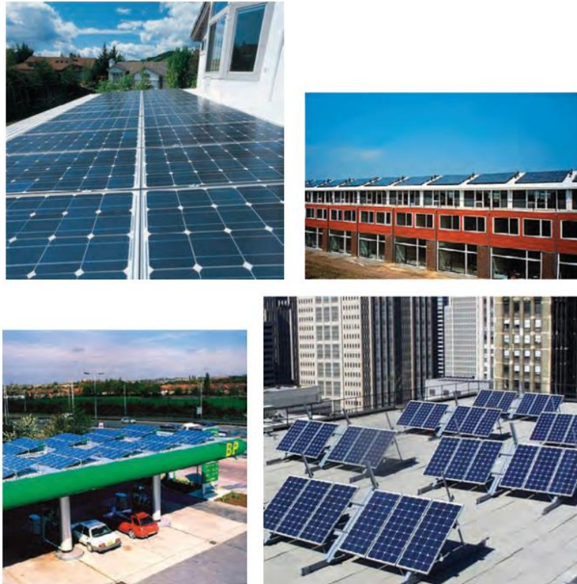
Figure 6.33 Various photovoltaic systems. (Image courtesy of the US Department of Energy, Washington, DC.)
