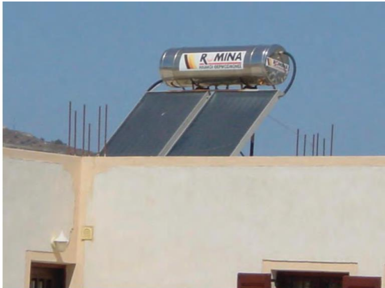
Figure 6.5 Passive thermosiphon hot water solar system.
