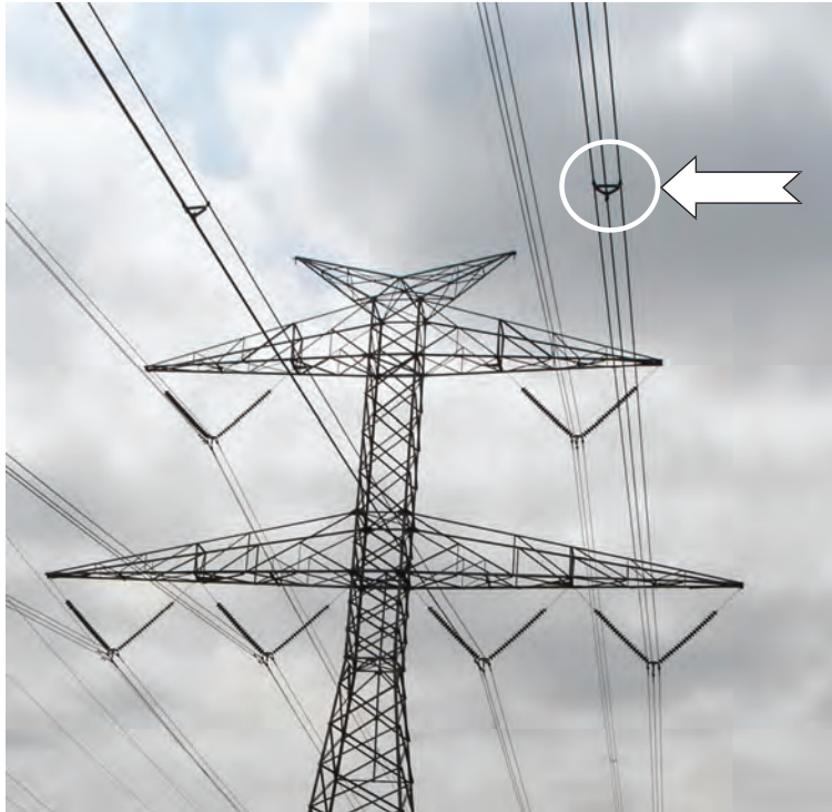
Figure 2.9 Bundled conductors.
