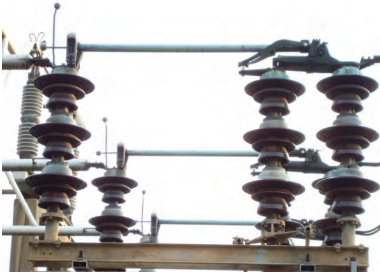
Figure 2.23 Disconnect switch.
