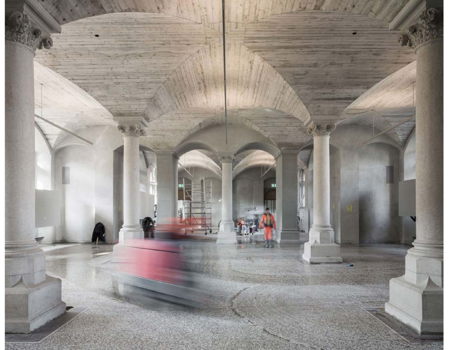
newly-cast concrete vaulted ceilings
