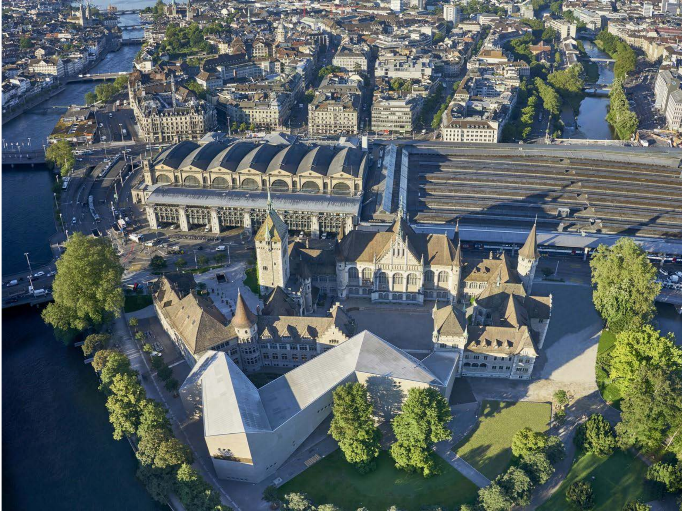
the origami roof of the new building - pitched roofs of the original.
