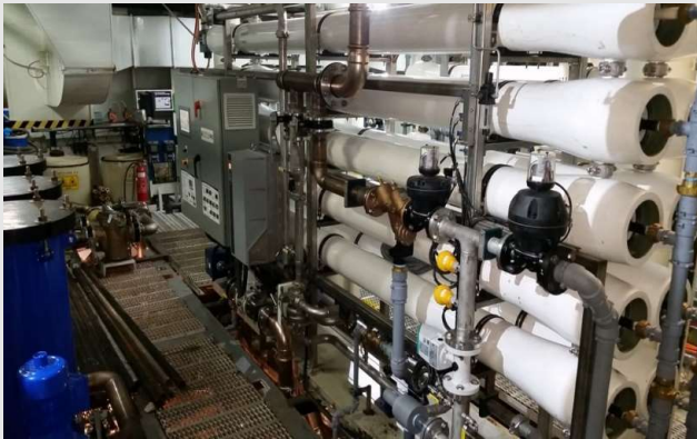
Reusing ballast water through desalination by reverse osmosis
