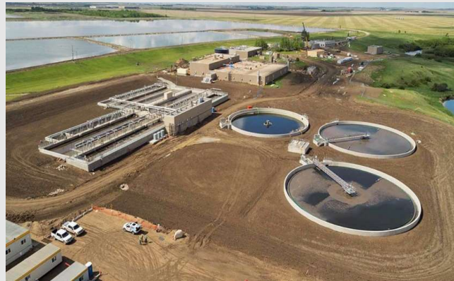
Onshore fresh water or municipal waste-water treatment
