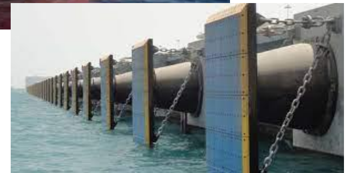
Fenders onboard and on the quay
