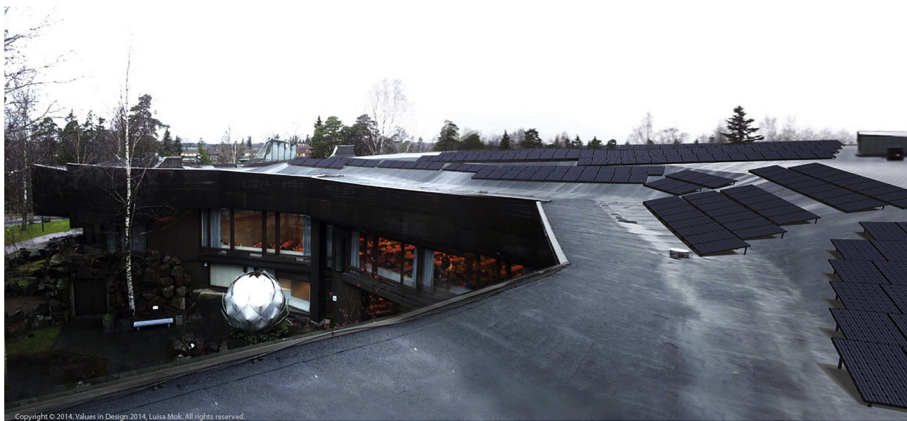
Figure 12 The solar array on the rooftop
