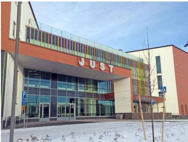
Järvenpää social and health centre "JUST" (completed in 2017)
