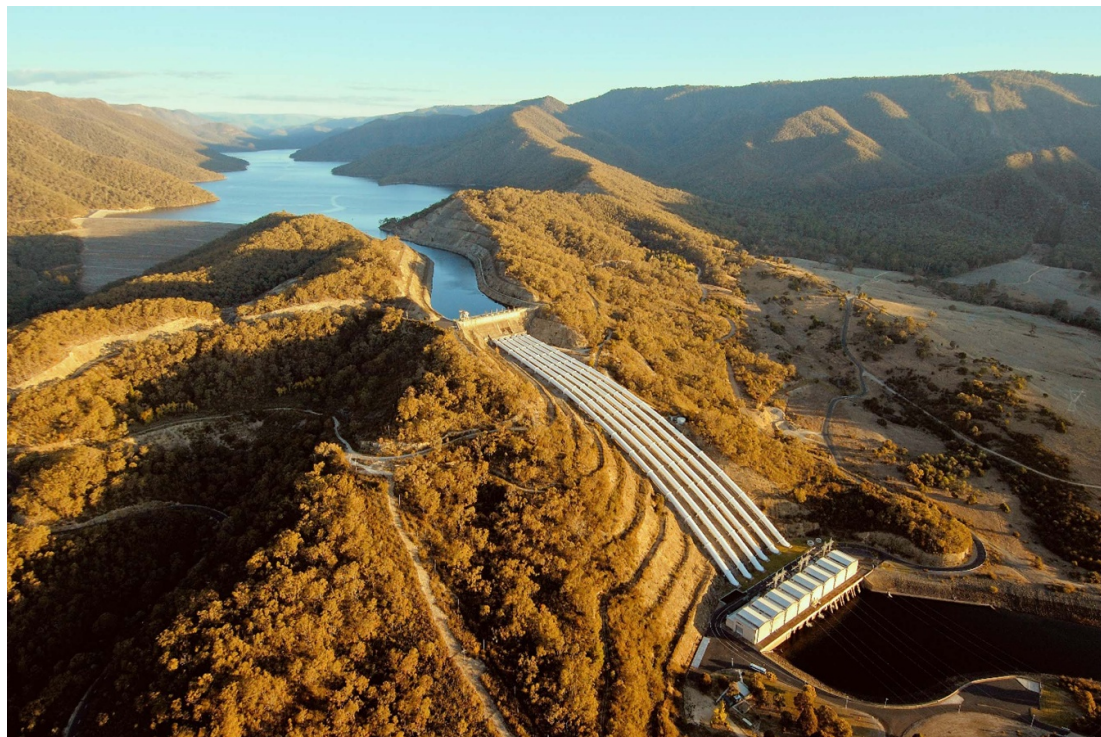
Figure 9. Tumut 3 on-river hydroelectric system (Snowy Hydro Ltd). Reproduced with permission from Snowy Hydro Ltd.
