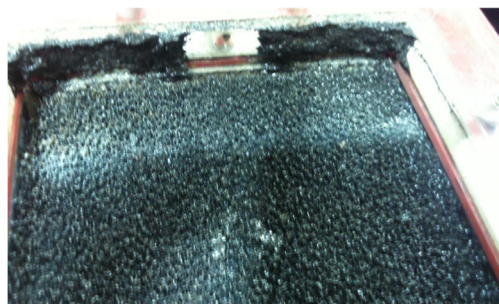
Fig. 6 Formation of sludge in the bottom of the electrolyte flow frames
