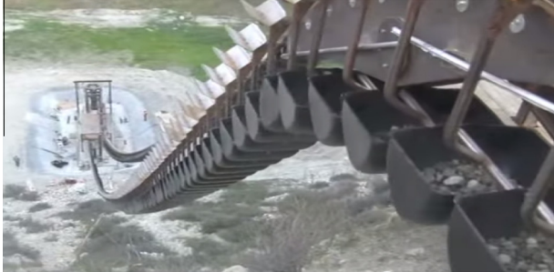
Fig. 11. Energy Cache 50 kW Gravity Energy Storage (ECGES) demonstration plant in California [36].
