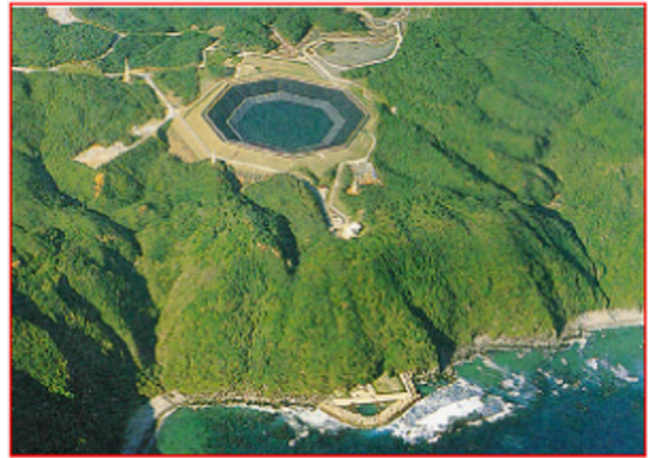
Fig. 8. Aerial view of Okinawa 30 MW capacity sea water pumped storage plant [133].
