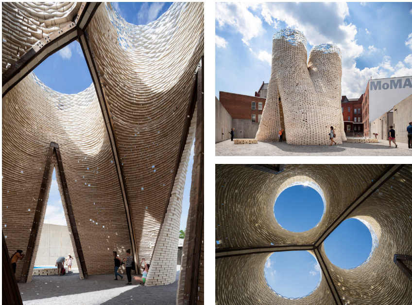
Hy-fi made by mycelium material The Living newyork studio Link: http://www.thelivingnewyork.com/
