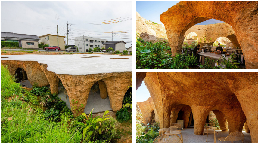
Mud -covered house & restaurant
