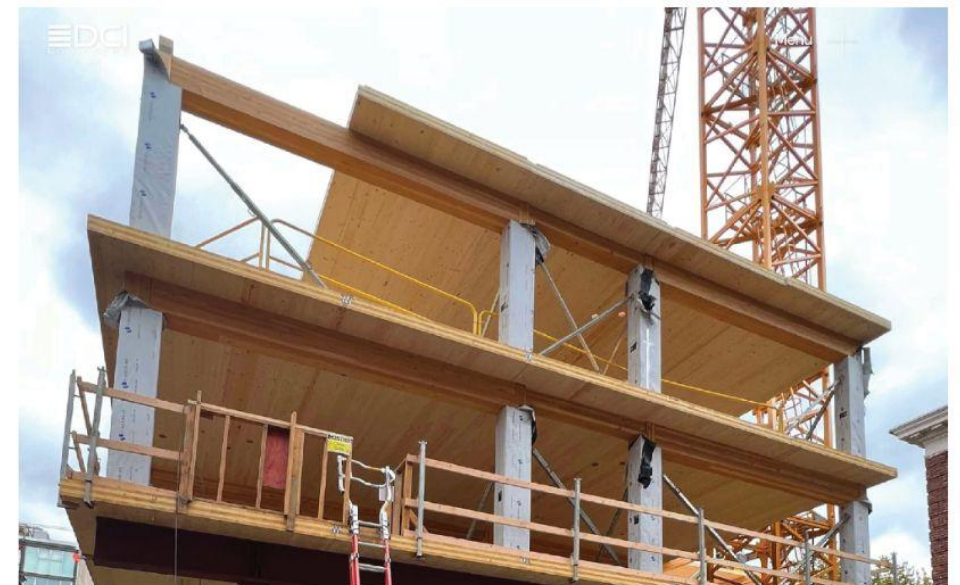
03 Site Photo of post-beam + deck installation
