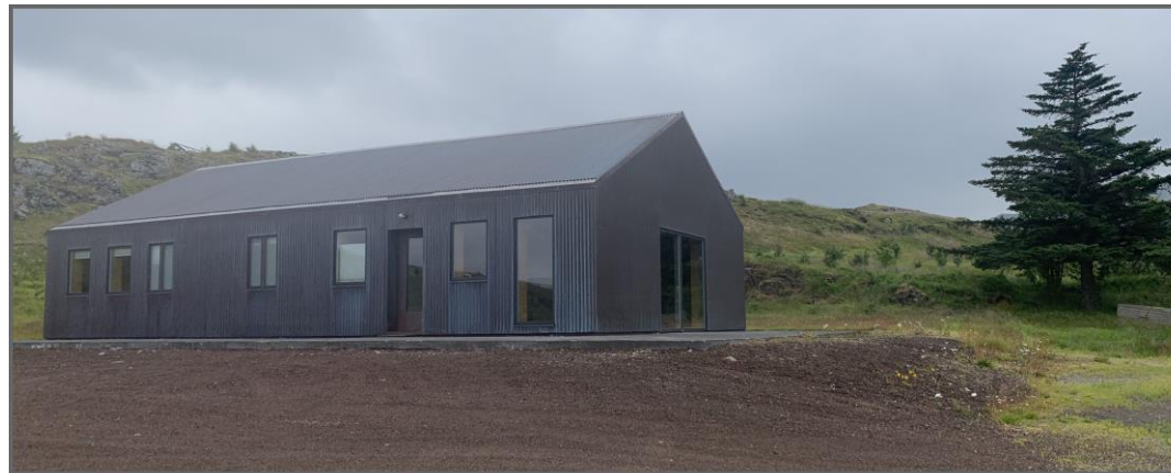
The former tractor shed
