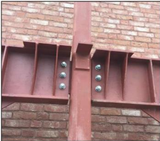
Installation of used steel on site. Photo: Stokke Stål
