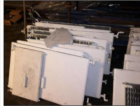
Storage before flushing and pressure testing. Photo: Anders Sand
