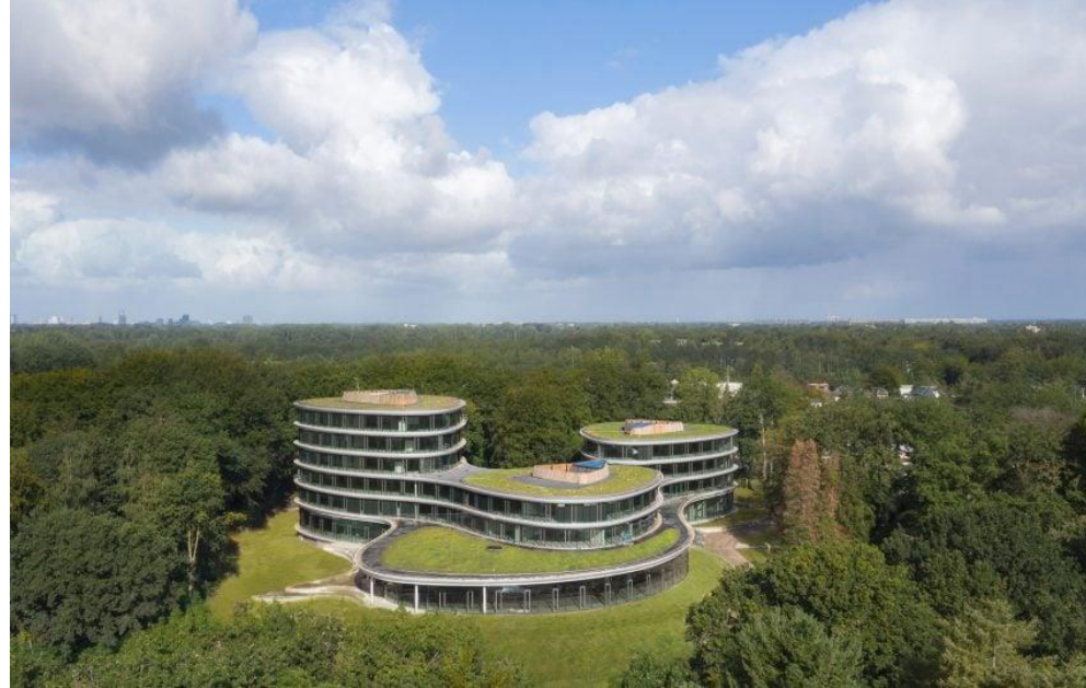
Triodos Bank office, Netherlands
