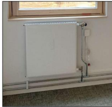
Complete assembly after processing. Photo: Randi Lunke
