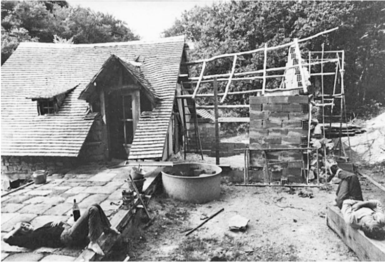
House under construction, La Vallée.
