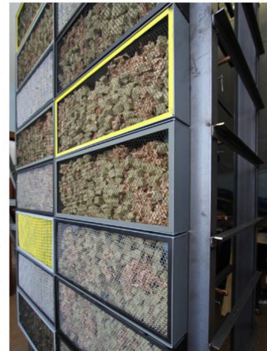
Richard L. Hindle, Plant Substrate of cubed mineral wool and long grained sphagnum moss retained by painted lath and folded sheet metal module.
