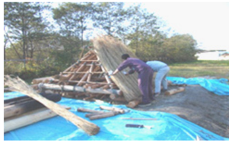
Construction of the roof
