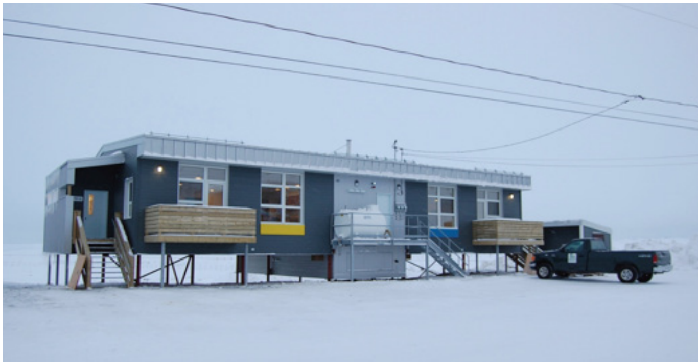
Figure 98. South facade of the prototype and simplified floor plan of the building. Société d'habitation du Québec ( www.habitation.gouv.qc.ca )
