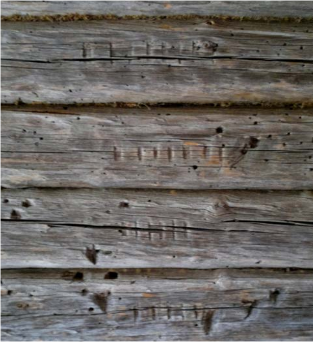
Figure 32. Transfer marks in the logs of a log house. Livady.
