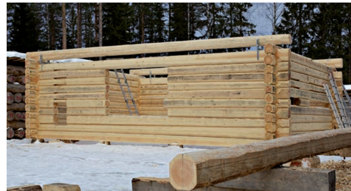
Figure 17. A log frame for a one-family house under construction. Livady .
