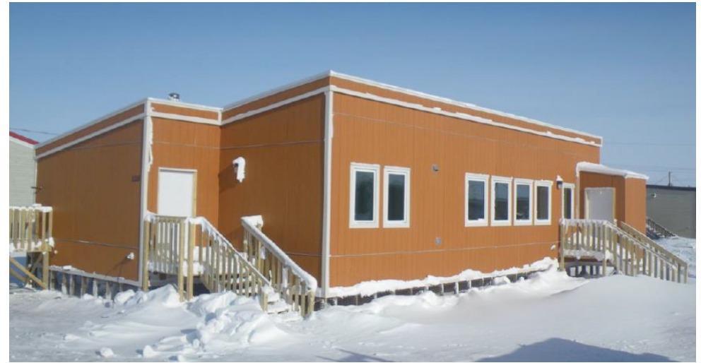
Figure 70. Arviat E/2 Northern Sustainable House (Nunavut). https://www.cmhc-schl.gc.ca/en/data-and-research/publications-and-reports/arviat-e-2-northern-sustainable-house-energy-consumption-performance-assessment
