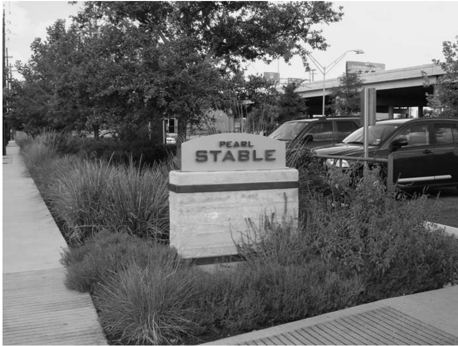
Figure 1. Rain garden implemented at the site perimeter at the Pearl Brewery redevelopment in downtown San Antonio, Texas, sufficient to ensure percolation of rain runoff. Design team included Rialto Studio, Lake|Flato Architects, Sprinkle & Company Architects, Three Architecture, Pape-Dawson Engineers, and Danysh & Associates Structural Engineers (Photo courtesy of Rialto Studio).
