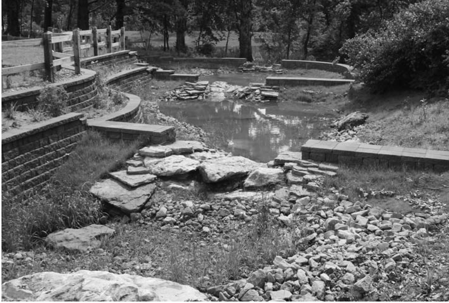
Figure 4. A series of bioretention cells captures and treats stormwater on site at the John Burroughs School in Laude, Missouri. Design team included Christner, Intuition and Logic, Volz, and John Burroughs School (Photo courtesy of John Burroughs School).
