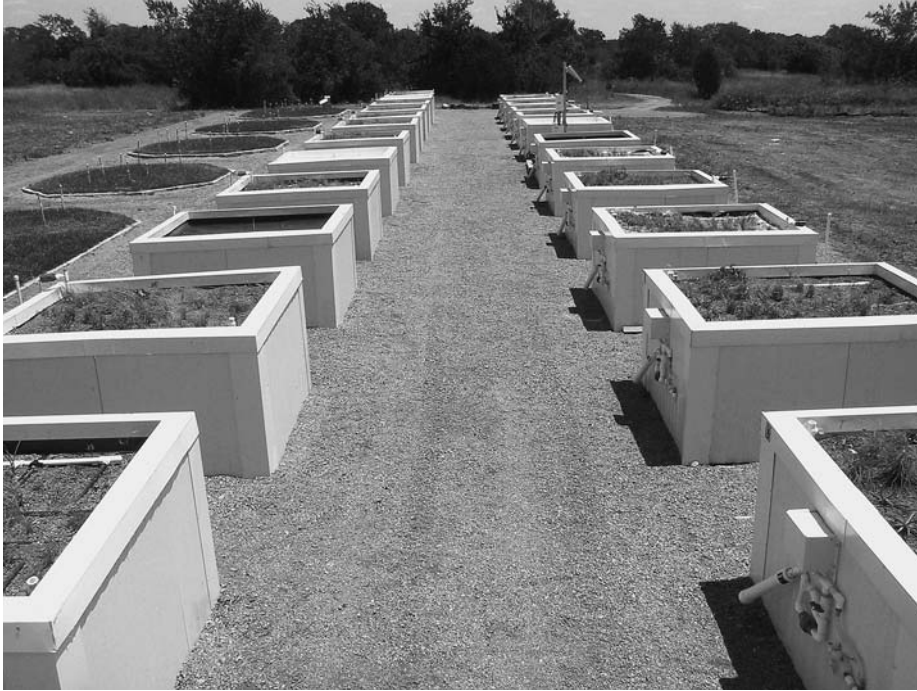
Figure 2. Green-roof research plots at the Lady Bird Johnson Wildflower Center, Austin, Texas. The study found significant differences in performance in terms of plant success, quality of water runoff, and water-detention capacity among six green-roof manufacturers (Photo by Mark Simmons).
