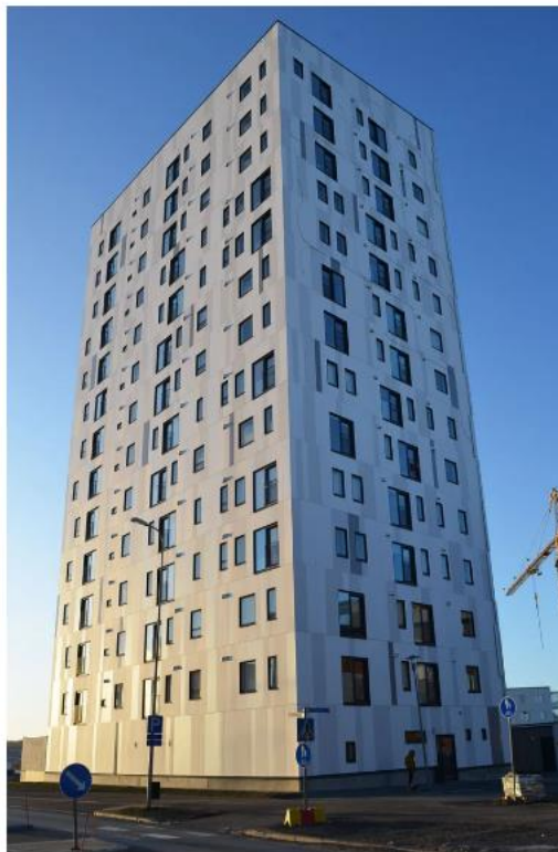
This apartment building in Joensuu is, according to its designers, the tallest all-wood building in the world.
