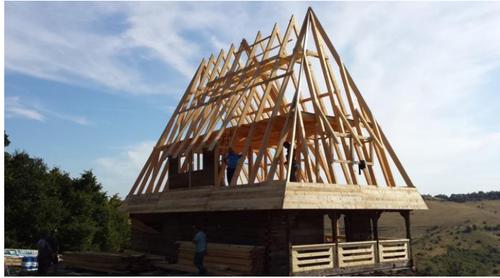
Relocated and Reused Ground Floor of Family House
