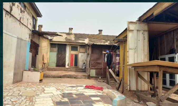
Typical detached compound house
