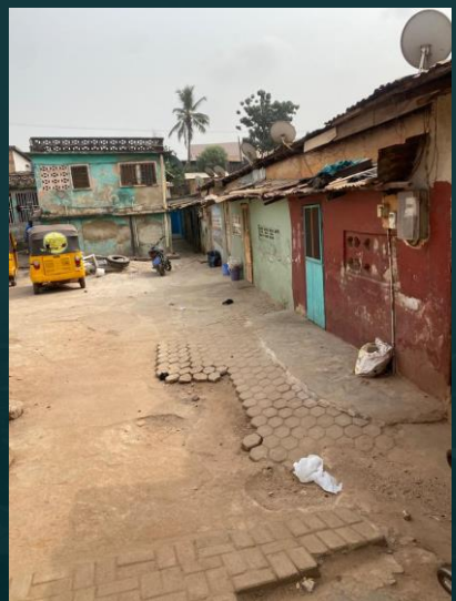
Typical detached compound house
