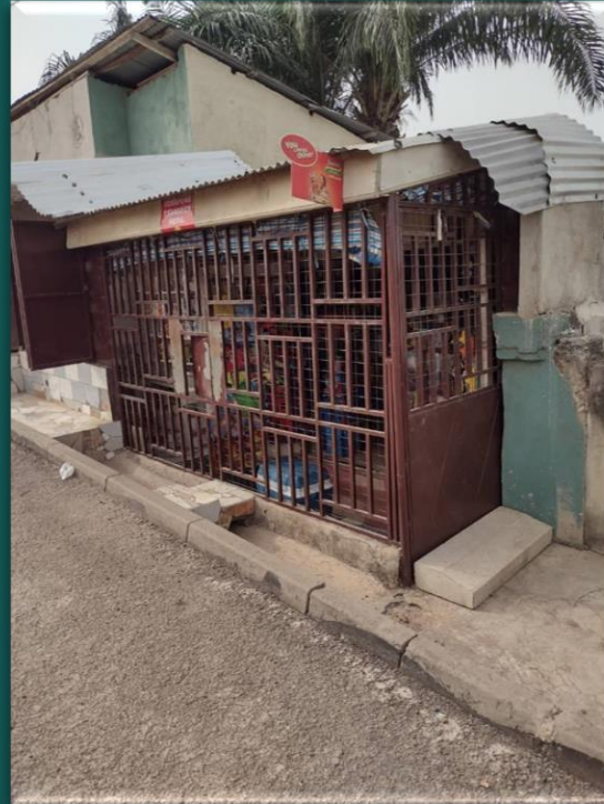
Image showing typical metal container store
