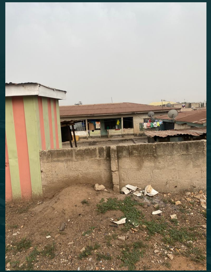
Typical detached compound house
