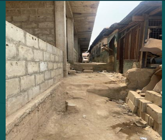
➤ Image showing unfinished corridor and staircase
