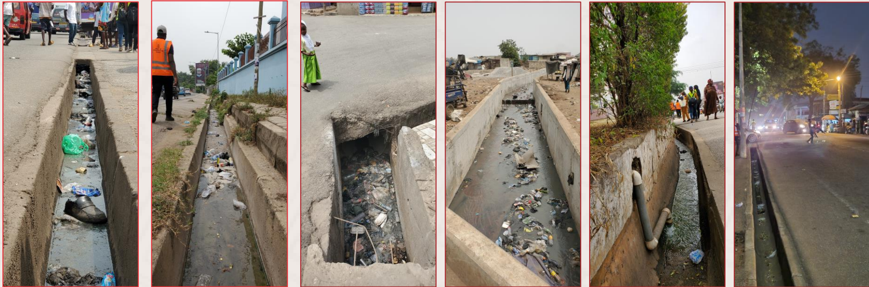
Images showing some major street drains for all the zones
