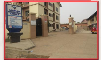
• Anwiam Hospital Annex SURVEY 2023
