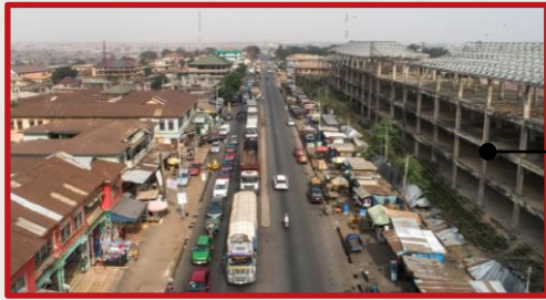
P.V. OBENG BYPASS ROAD
