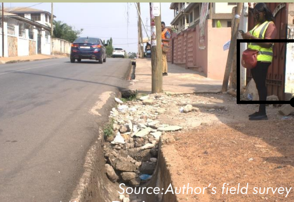
Source: Author's field survey Minor Drains Lat: 6.709366 Long:-1.612248
