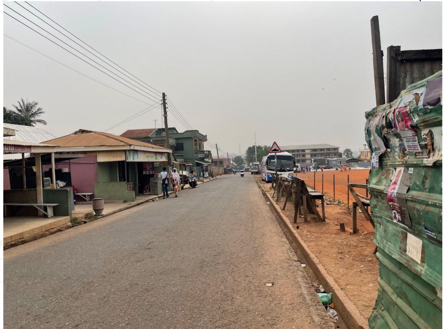
View of Asare Drive streetscape
