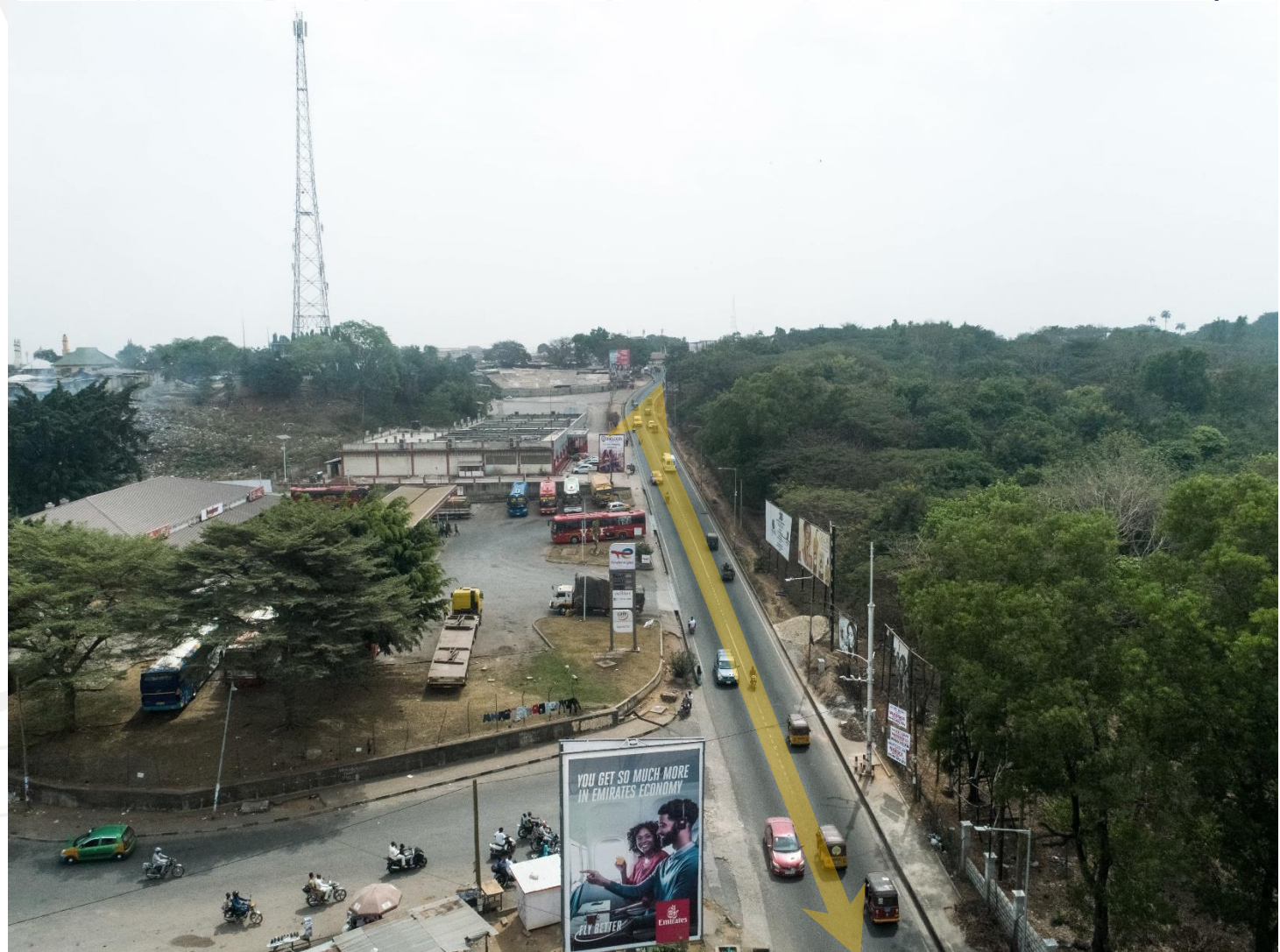
Aerial view of Antoa/ Manhyia Road towards the Manhyia Roundabout.
