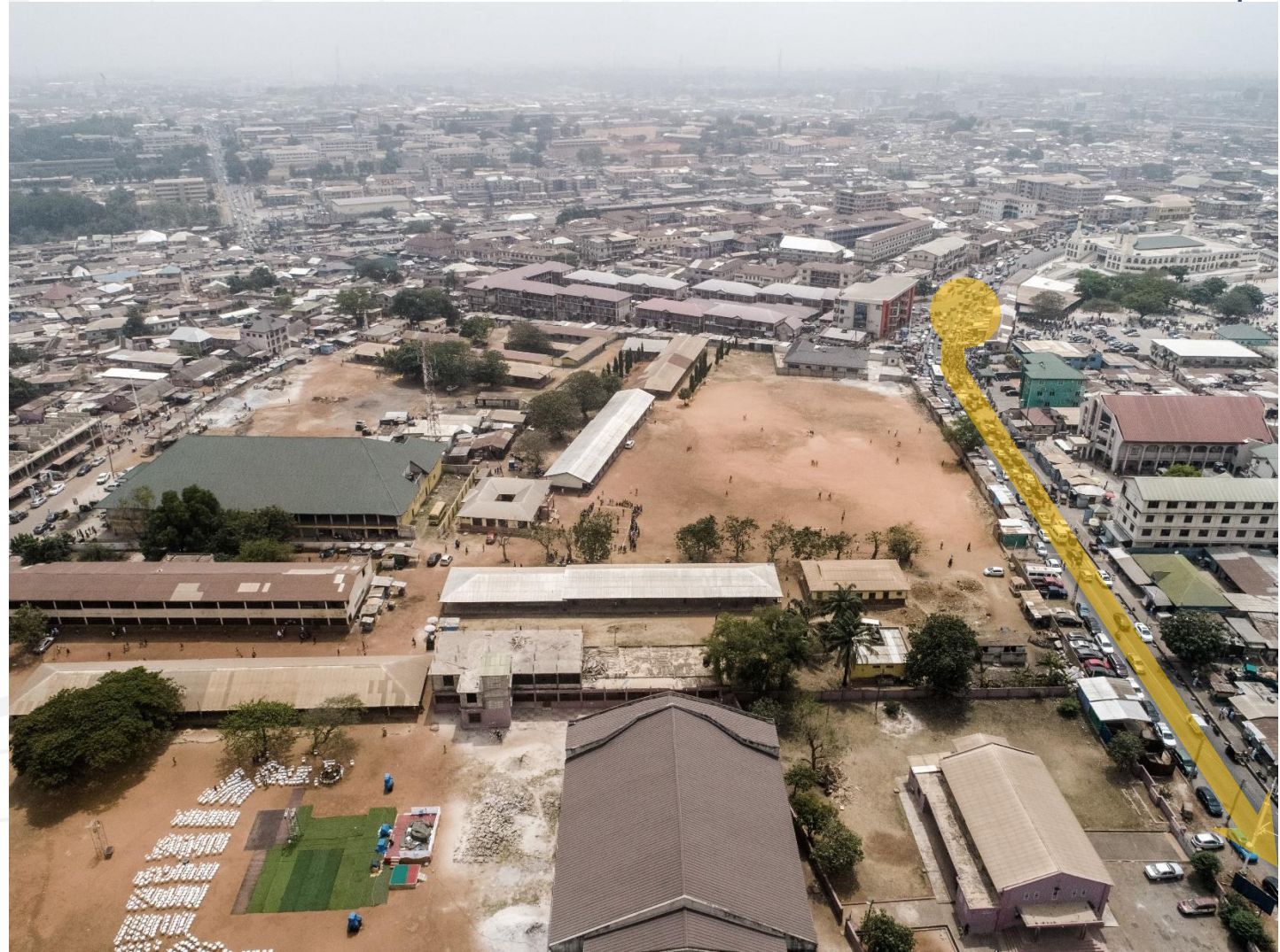
View of Burma Road towards the Central Mosque
