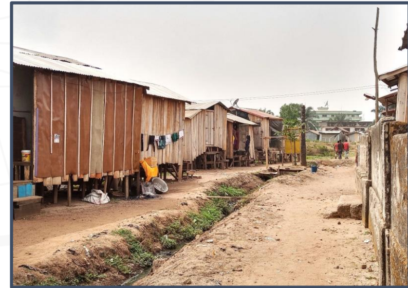
Slum development in and around the focus areas, raised buildings to prevent flooding of the structures which serve as shops and residences. Source: Urban Field Study - 2023
