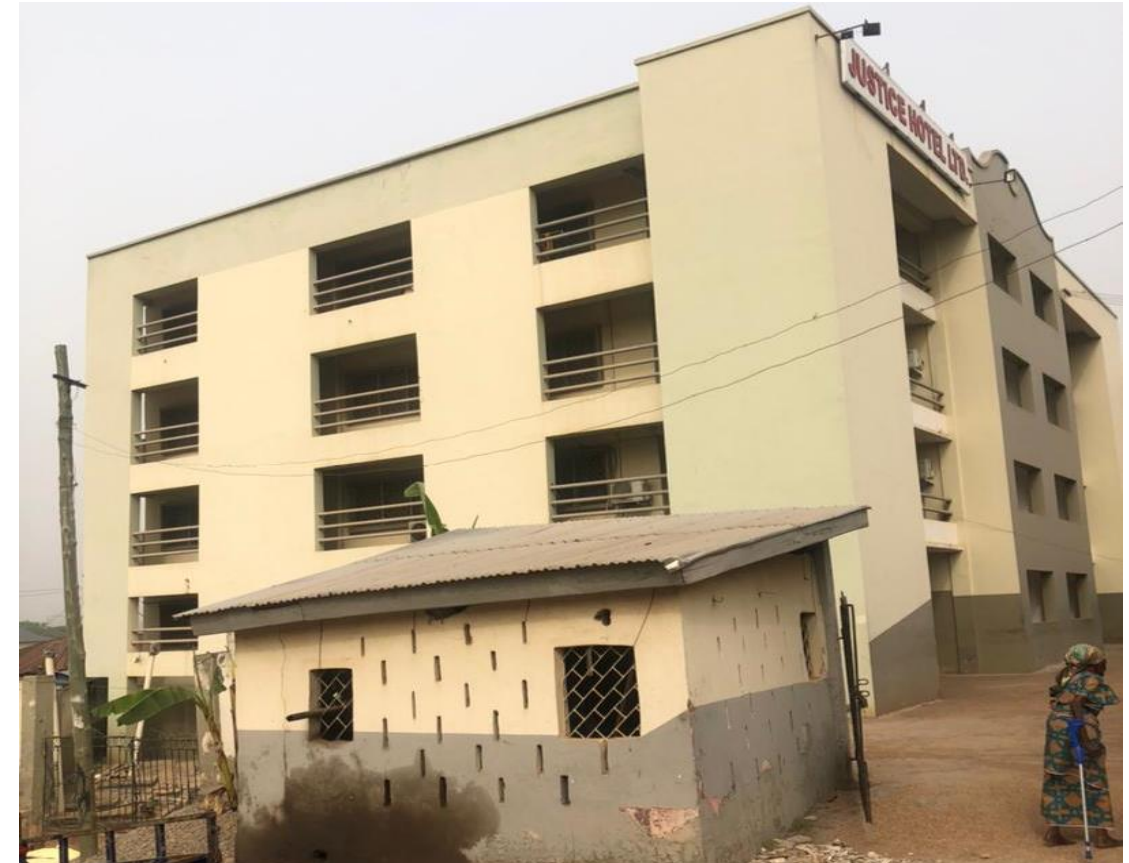
A renovated building in zone 4
