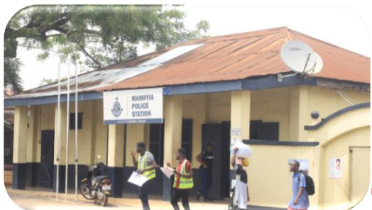
Manhya Police station
