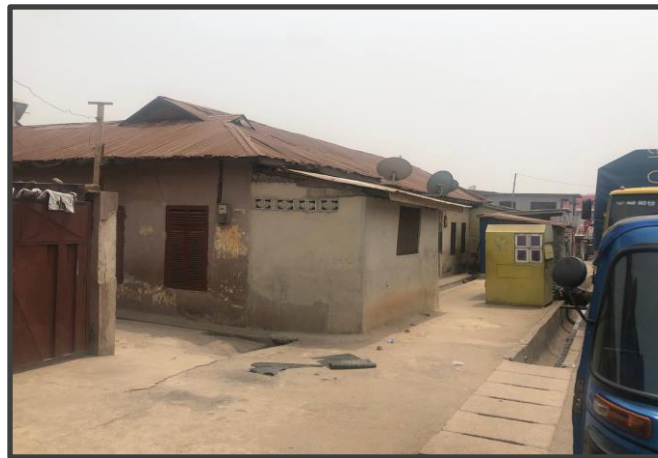
Old building with Extension built with sand crete
