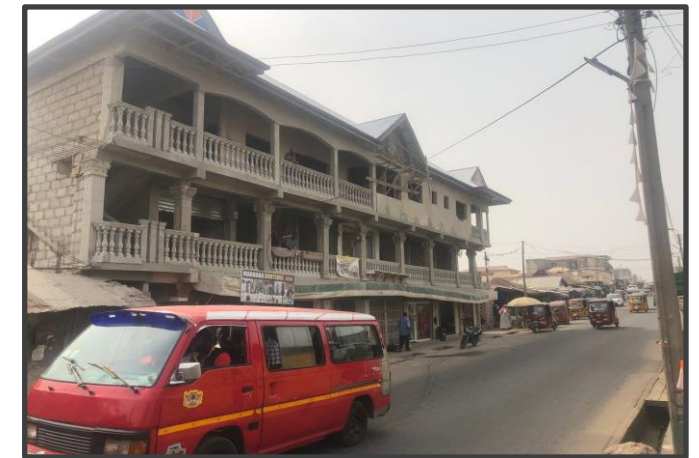
New building built with sandcrete blocks
