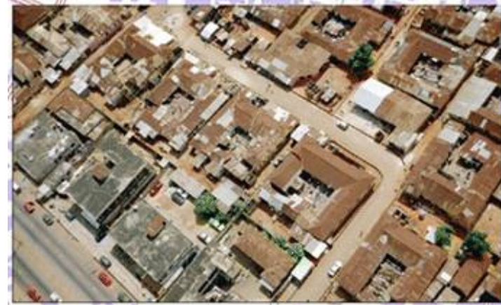
Unauthorized building extesions
