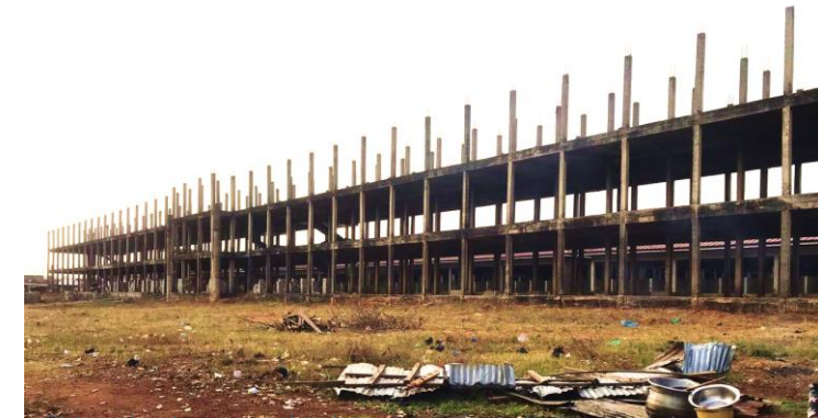
Picture showing uncompleted structures of new Krofrom market
