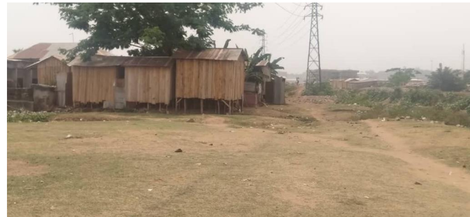
Unauthorized building extesions
