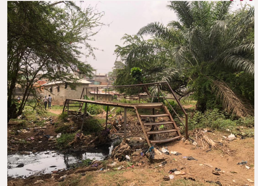
Bridge access to school facility
