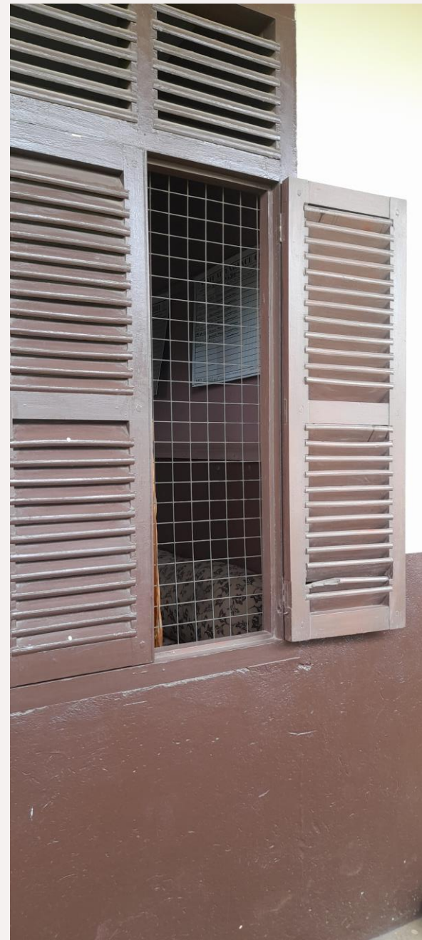
Wooden shutters for ventilation
