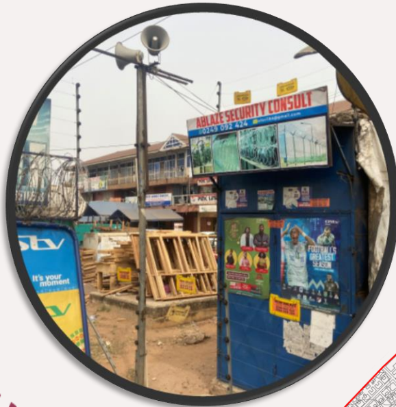
P.A system on steel pole
