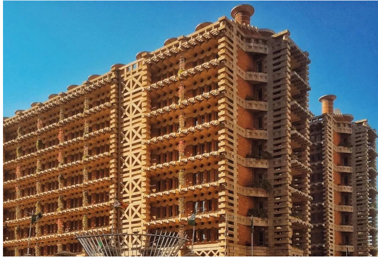
Passive cooling system inspired by termitier Eastgate Centre, Harare, Zimbabwe, Mick Pearce, 1996
