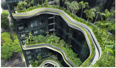
Green roofs & skins
