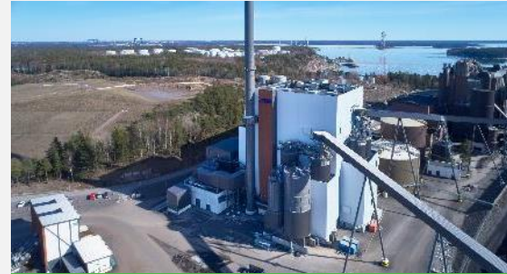
Multifuel to energy
