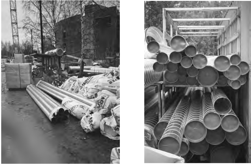
Figure 3.21 Air ducts at a construction site (left) can cause considerable air pollution indoors after installation, caused by accumulated dust/debris; capping the ducts (right) is a good solution
