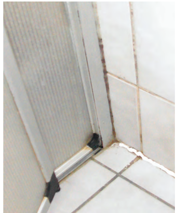
Plate 5 Mould growth in shower cabins almost always occurs on the water-resistant sealant
