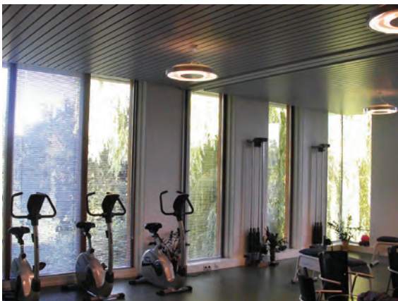
Plate 4 Integration of daylight and artificial light: In this situation the solar blinding placed on the inside of the glazing is not efficient at remedying overheating caused by solar radiation
