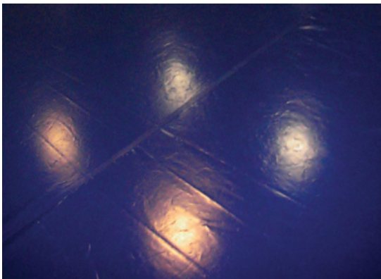
Plate 3 Reflections of ceiling lights on a shiny smooth floor: This situation can cause enormous eyestrain
