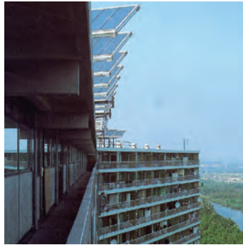
Plate 19 Solar collectors on the roof of an apartment building
