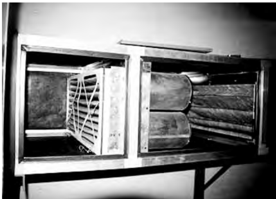
Figure 3.27 A multi-stage filtering system that features an absolute active carbon and a filter bag
