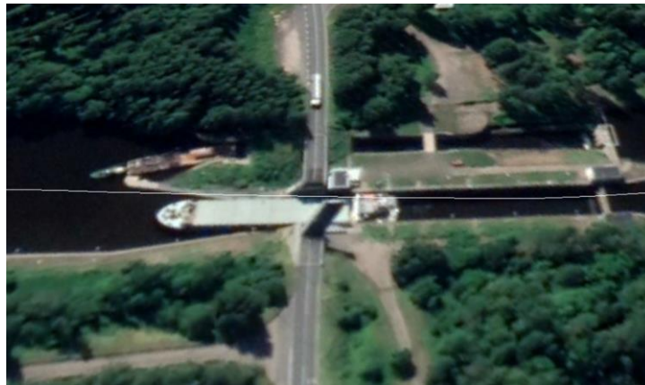
Figure 2 bascule bridge while a cargo vessel passes through
