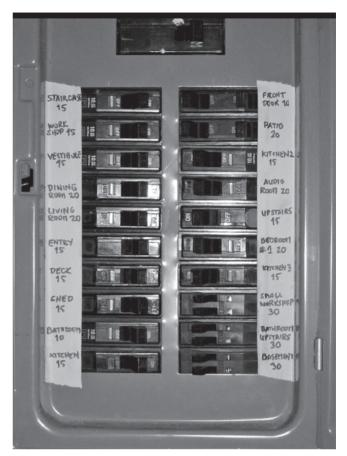
■ Figure 18-12 Electricity on location. A lighting crew has carefully labeled this household breaker box after determining where each circuit is located and what the amperage rating is.
