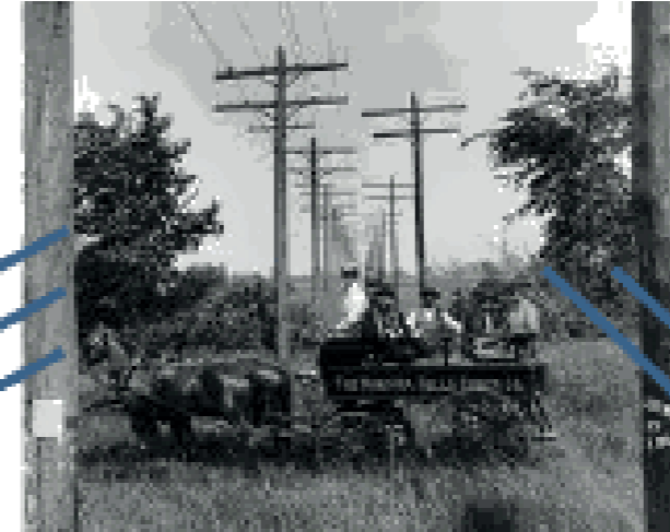
High voltage Transmission Lines
