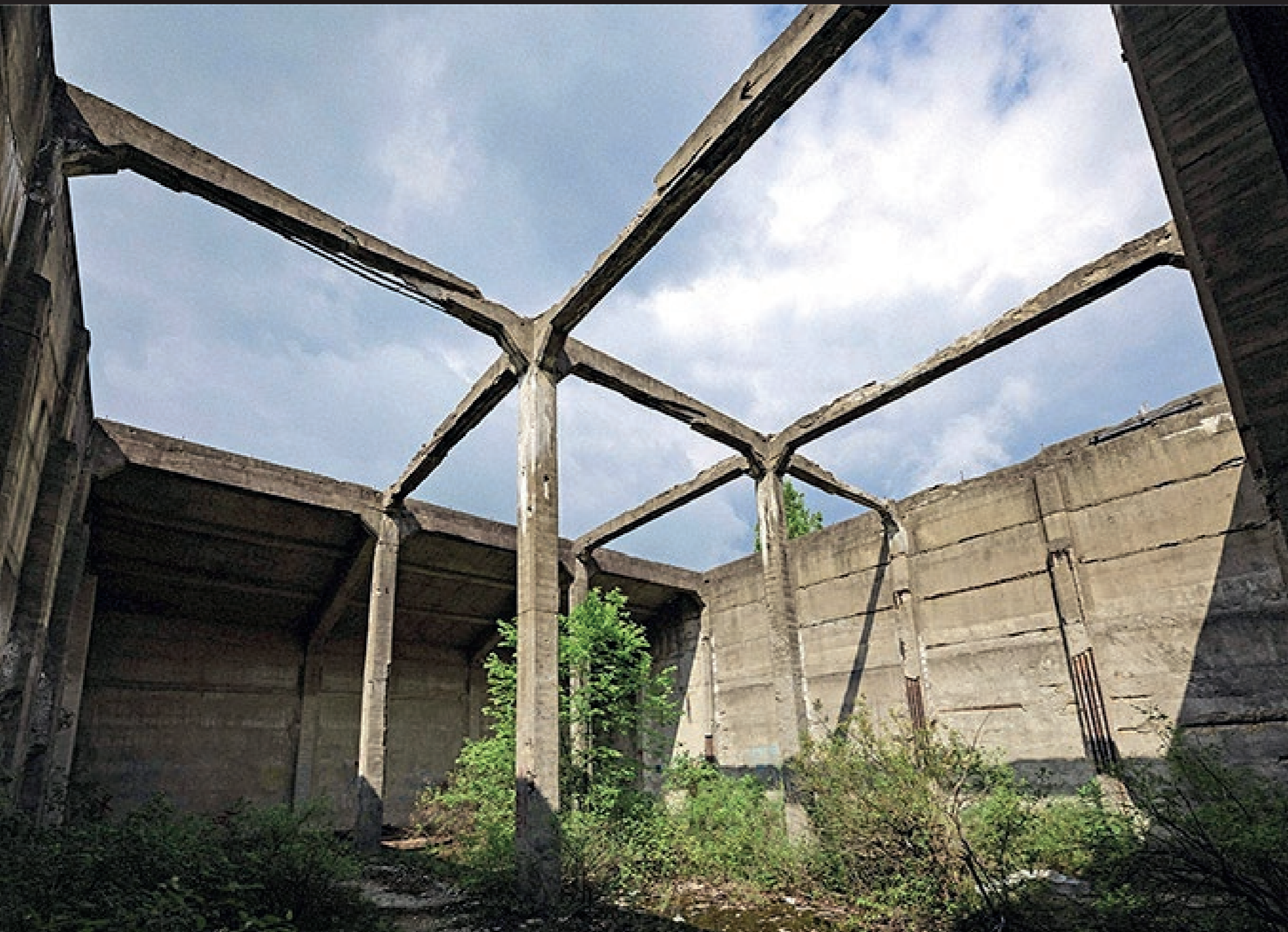
Great Northern Cement Company warehouse James Road, Marlboro, Michigan, 1904
