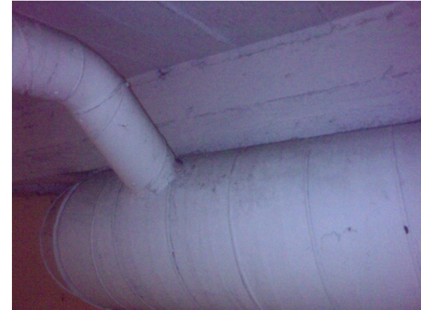
Perpendicular joint should be rounded
