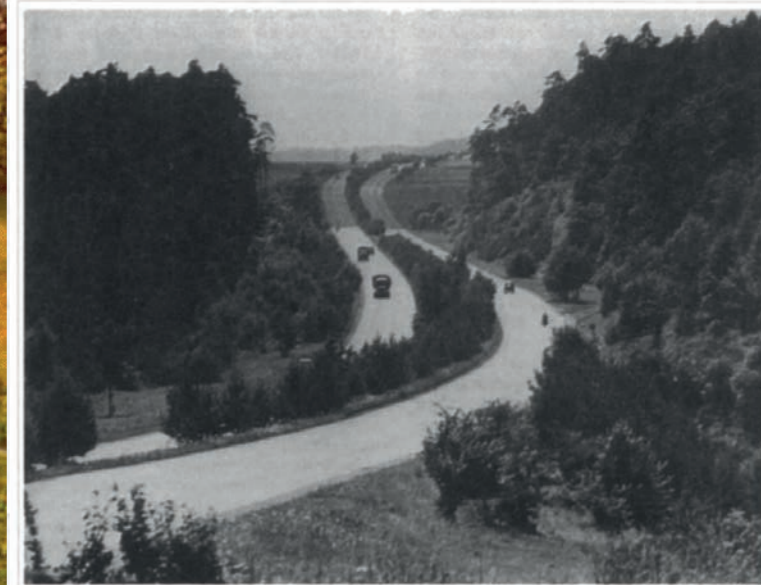
Figure 3. Section of the Autobahn between Frankfurt and Kassel, showing use of sinuous curves to fit the landscape and brushy plantings of local firs on the median strip. Crowe 1960: Figure 72.
