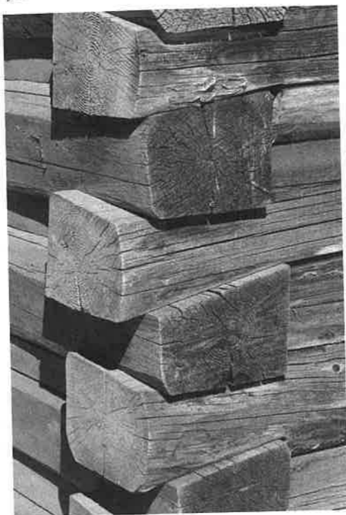
Figure 5.1 Joining timber. This photo, taken in British Columbia, Canada, illustrates one way of joining beams at the corner in traditional log-cabin construction. © Alex Fairweather / Alamy.
