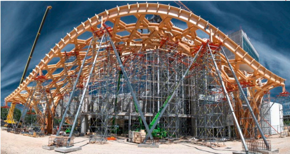
Figure 4. Shigeru Ban, Centre Pompidou, Metz, France, 2010
