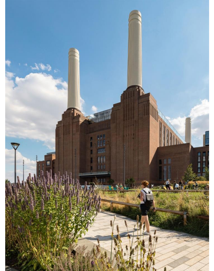
Battersea Power Station, London, WilkinsonEyre
