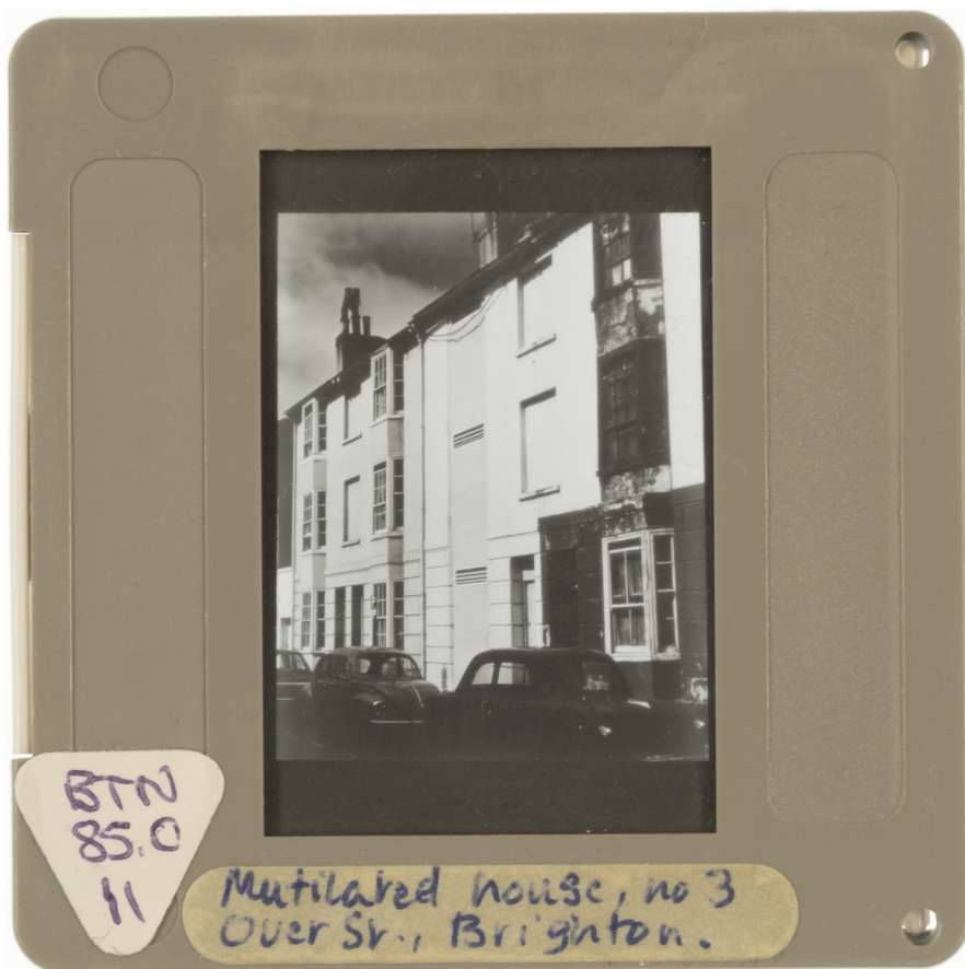
Figure 11. 'Mutilated house, No. 3 Over St, Brighton', undated 35mm slide, photographer unknown, former University of Brighton slide library, collection of Annabella Pollen. Photograph by Rachel Maloney, 2021.
