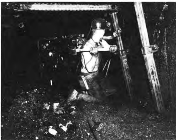
Figure 30. Miners installing roof supports.
