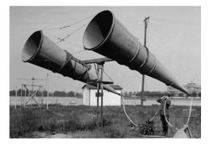
Binaural hearing was cost-efficient and accurate in detecting of direction of incoming aircraft
