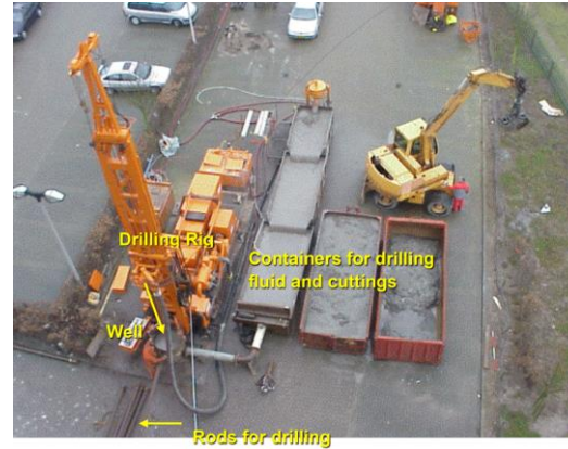
Drilling rig in action
