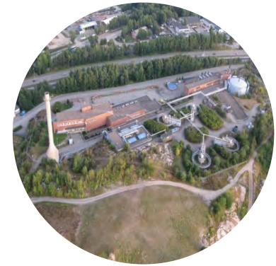
Viikinmäki wastewater treatment plant
