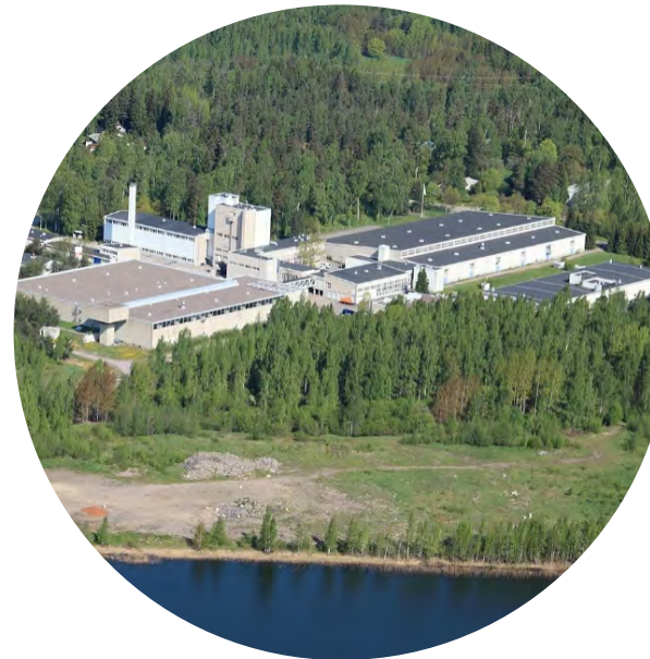
Pitkäkoski water treatment plant
