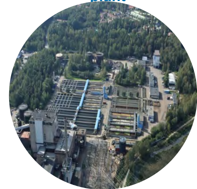
Suomenoja wastewater treatment plant
