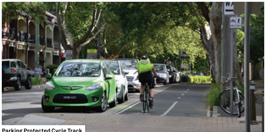
Parking Protected Cycle Track
