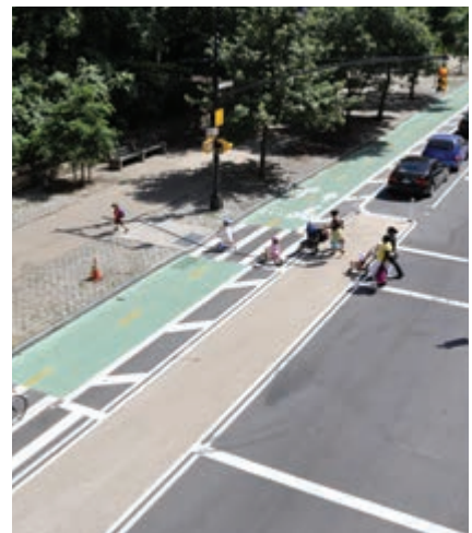
New York City, USA. A two-way cycle track along the western edge of Prospect Park.
