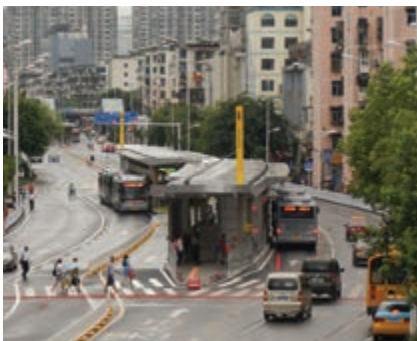
Guangzhou, China. This BRT system opened in 2010 and travels in a dedicated transitway.
