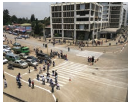
Addis Ababa, Ethiopia. An interim transformation showcasing the principles such as tightening the corner radii, adding appropriate intersection distance markings and reducing crossing distances.
