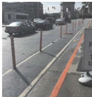
Flexible bollards delineate an interim bike lane.
