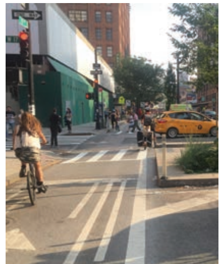
New York City, USA. A pedestrian refuge island and green infrastructure strategies are aligned with the parking lane, reducing crossing distances and increasing the safety of the intersection.
