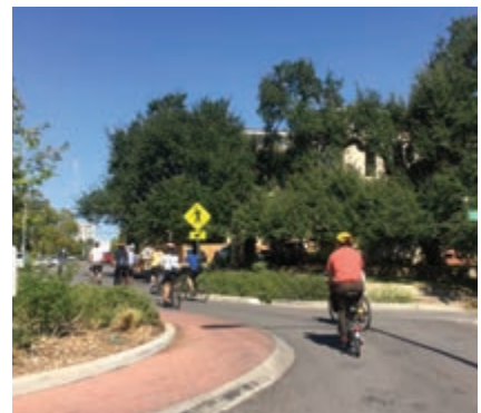
Austin, USA. A mountable curb in a neighborhood roundabout allows larger vehicles to navigate the intersection when required, while calming everyday traffic.
