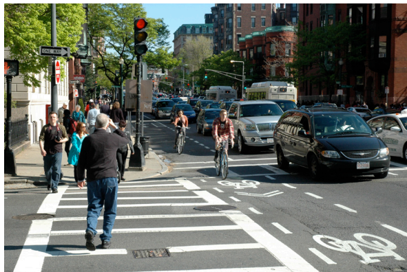
After Road Diet: Massachusetts Avenue with one parking lane, two travel lanes in each direction, and bicycle lanes in each direction, as well as transit prioritization at specific locations along the corridor.
