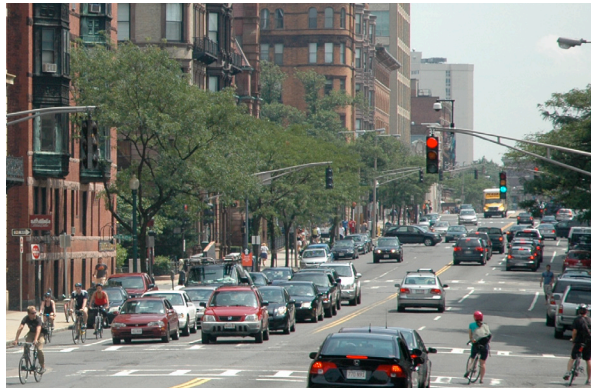
Before Road Diet: Massachusetts Avenue with parking on both sides of the street and two travel lanes in each direction.
