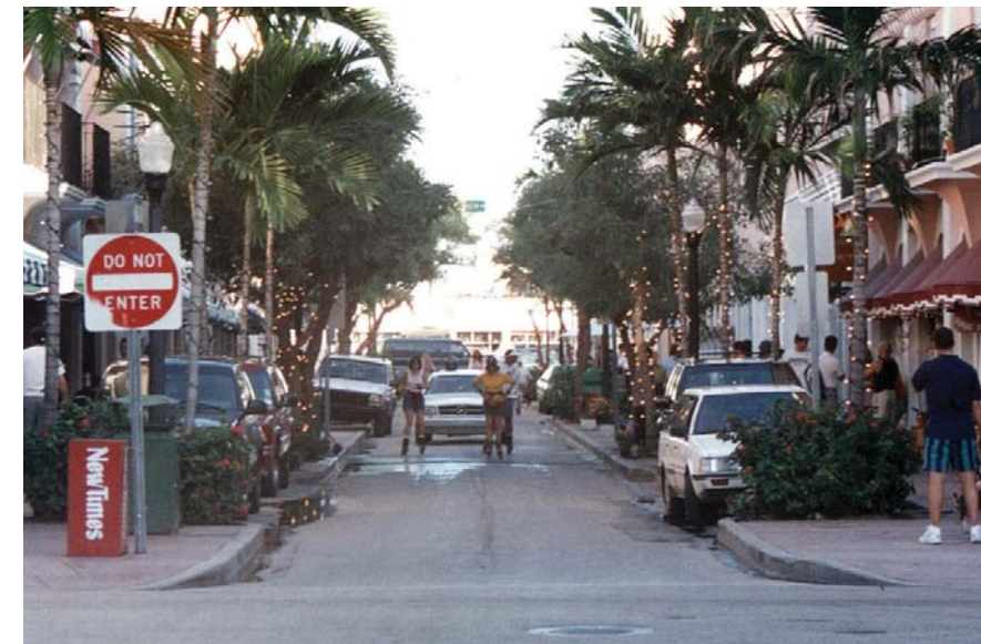
▲ Curb extensions shorten crossings and can act as a choker, narrowing traffic lanes at intersections to calm traffic, improving pedestrian safety at crossings
