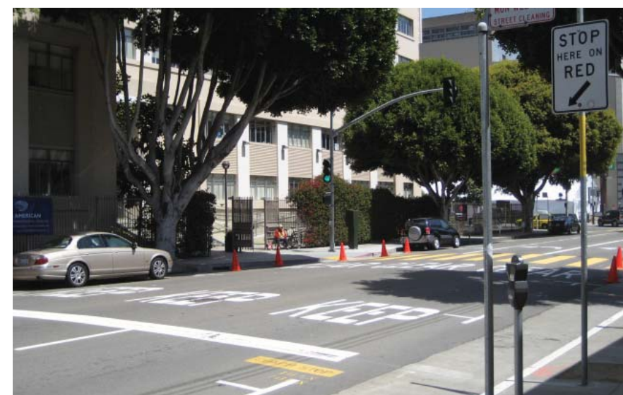
▲ Advance yield lines (top) alert drivers to an impending crosswalk; advance stop lines (bottom) require vehicles to stop in advance of a crossing
