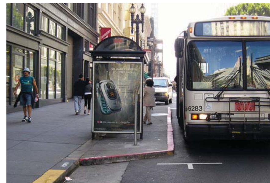
▲ Bus bulb-outs improve transit performance by allowing transit vehicles to load from the travel lane.
