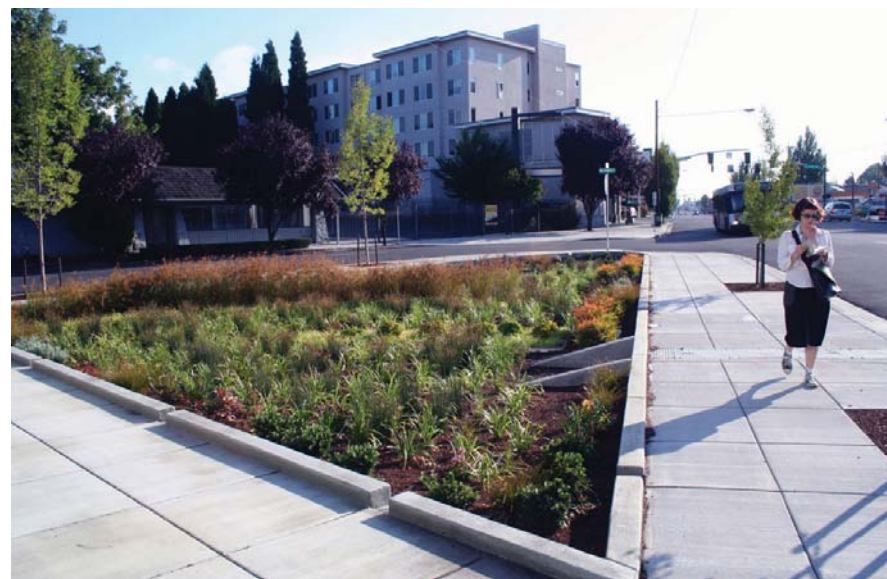
▶ Rain gardens are highly customizable, and can be designed to fit into any number of spaces within the streetscape. This raingarden includes a channel, behind the pedestrian, to convey roadway runoff to the landscaped treatment area. Source: Kevin Perry
