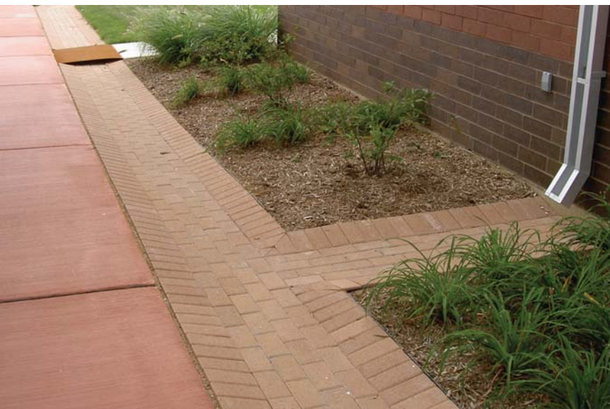
▲ Channels and runnels direct water through hardscape features to other stormwater management facilities
