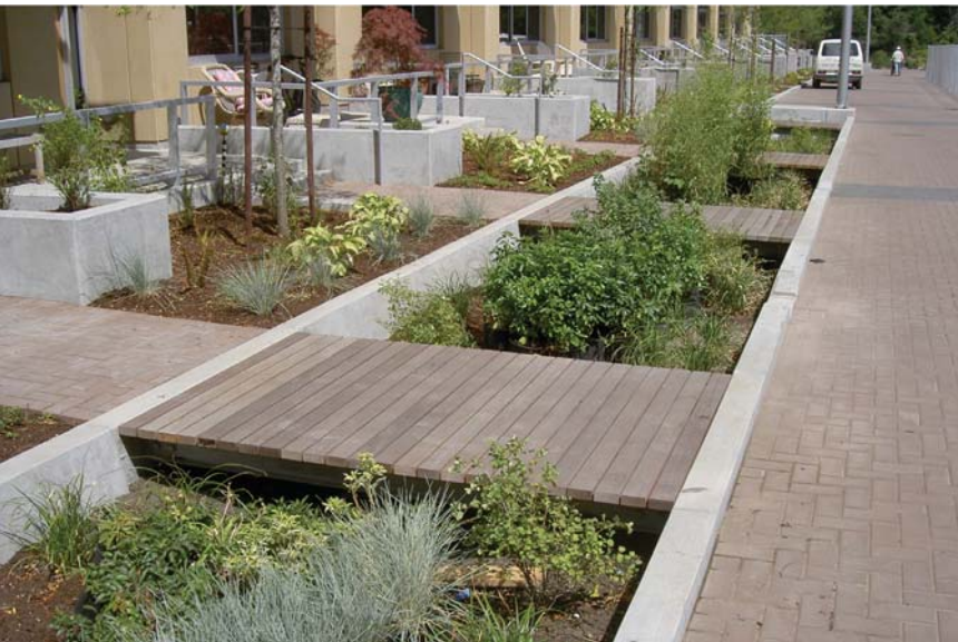
▲ This apartment building uses boardwalks over an infiltration area to define unique entrances to each unit from a shared public way Source: Sherwood Design Engineers
