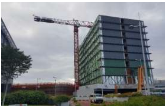
View of site from Terminal 2 during PPVC module installation
