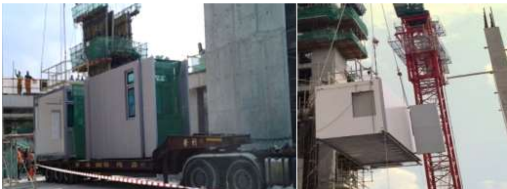
Delivery and hoisting of PPVC module on site
