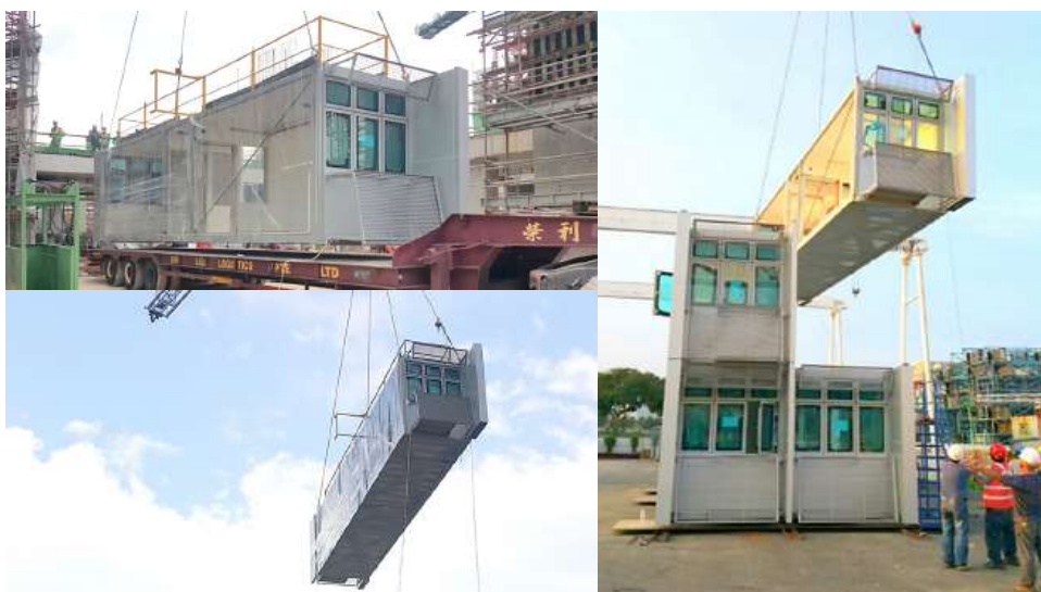
Fabrication of the PPVC modules (Images source: Singapore Piling & Civil Engineering)
